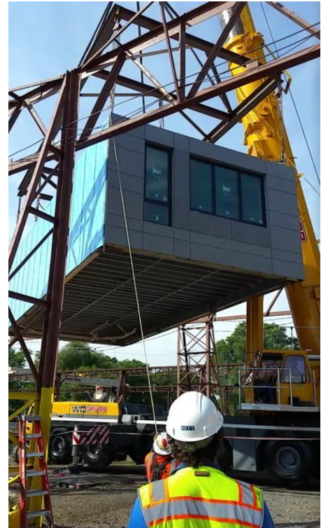
Photograph 7. Modular unit being hoisted onto the building
